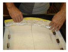
17. Reinstall the insulation with the foil side facing the inside of the broiler.
